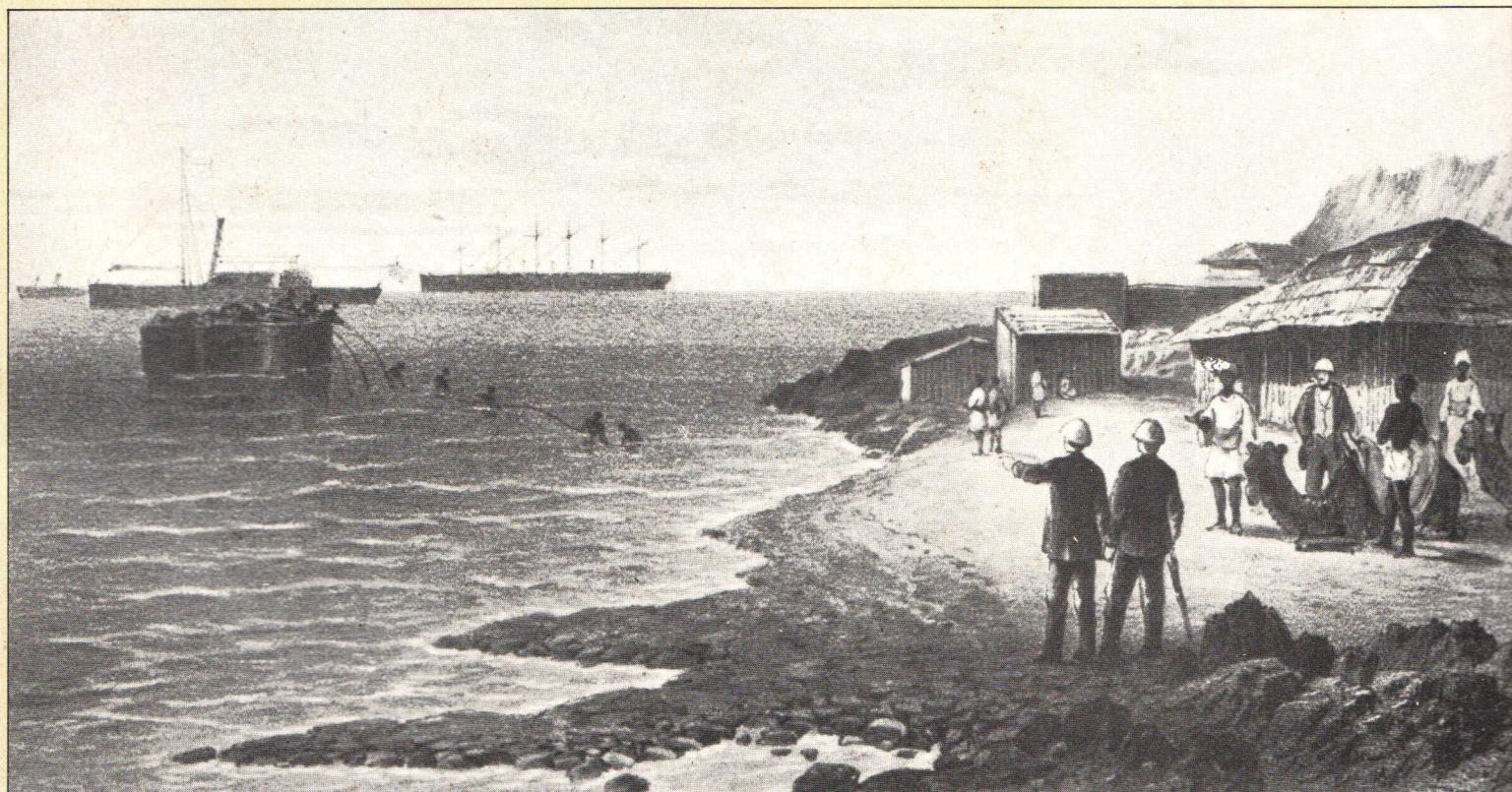
The Great Eastern lies off Aden's volcanic shores after laying the ocean telegraph from Bombay in 1870. In the foreground Arab workmen land the cable from a barge on the last stage of its journey to the telegraph office.
